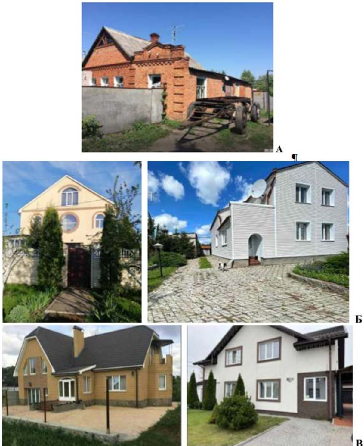
Figure 4. Examples of residential construction in different zones.
